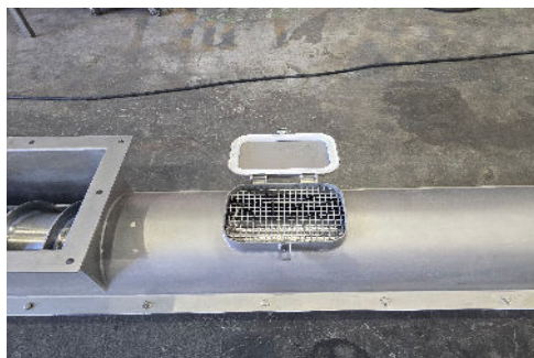
Inspection Port Located Downstream of Inlet
