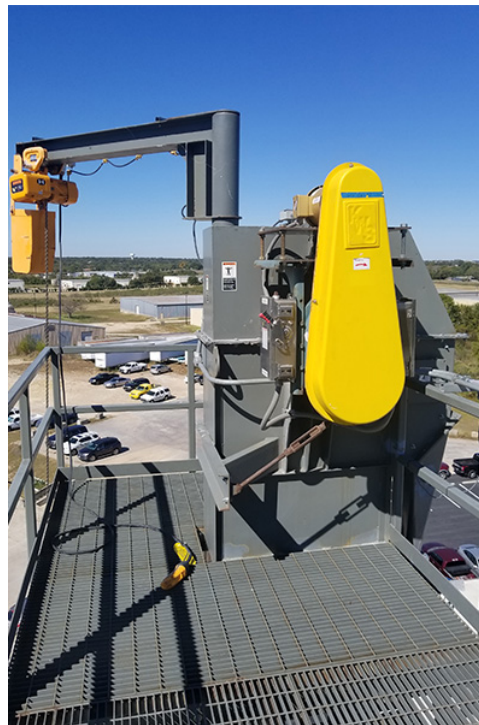
Jib Cranes Assist in Lifting Heavy Components to Head Section
