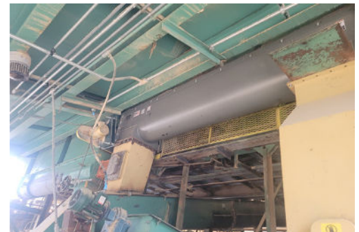
Accurate Field Measurements Made Installation of New Screw Conveyor Very Easy
