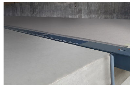
Multiple Inlets were Located Along Full Length of Screw Feeder
