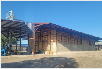
New Storage and Load Out System was Needed for Added Capacity
