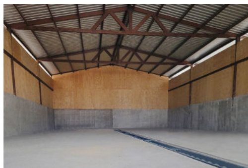
Floor Screw Feeder was Very Important to Success of Project
